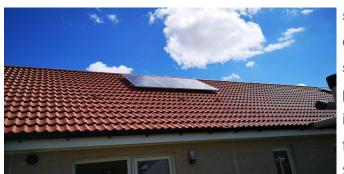
sunlight into electricity to use free of charge within your home. A solar PV system is made up of a number of panels connected together with an inverter. The type of system we have fitted to your home is roof mounted. Solar PV can still generate some
