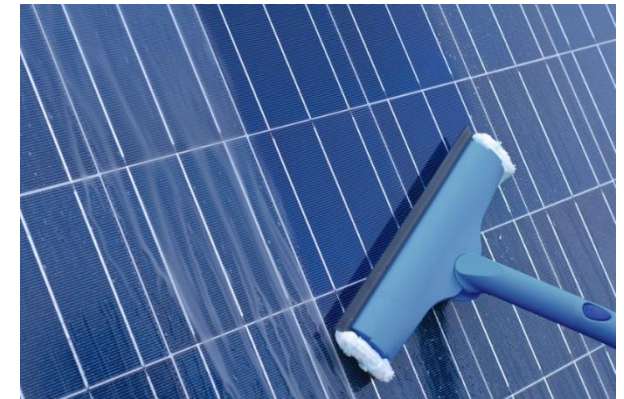
↑ Above: Solar PV panels require washing once a year to maintain efficiency
