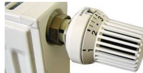
↑ Above: TRV's installed in each radiator
