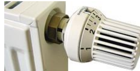
↑ Above: TRV's installed in each radiator
