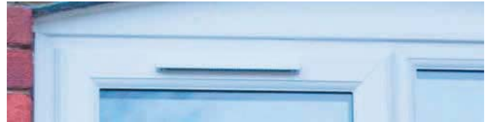
↑ Above: CMS windows with trickle vents (external view)
