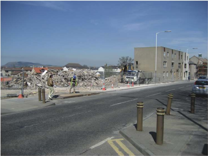
Main Street, Lochgelly. Buildings demolished for new build.
